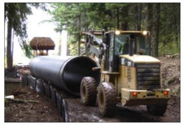
Commencing in November 2003, the project consisted of over 4,800 feet of 72" RSC160 Weholite Pipe and 25 mitered elbows with on-going earth ditch replacement under consideration.
